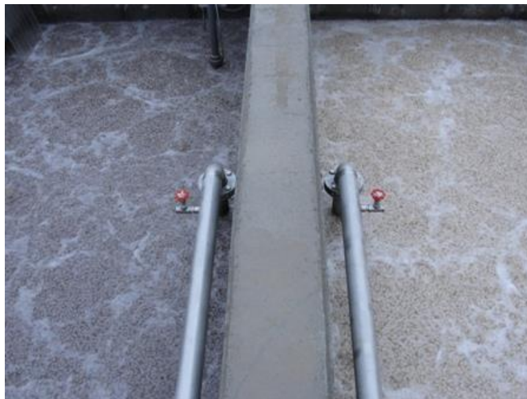
Figure 4 MMBR system in operation (media movement with aeration)
